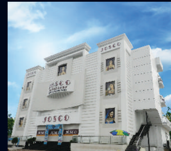
Tee Cee Commerce Gate, Thodupuzha. Actual Project
